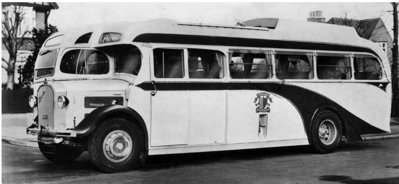
Harry Graveling acquired this 1937 Dennis Lancet registered CVC 700 circa 1953 and the chassis carried a thirty-two seat Willowbrook body.
